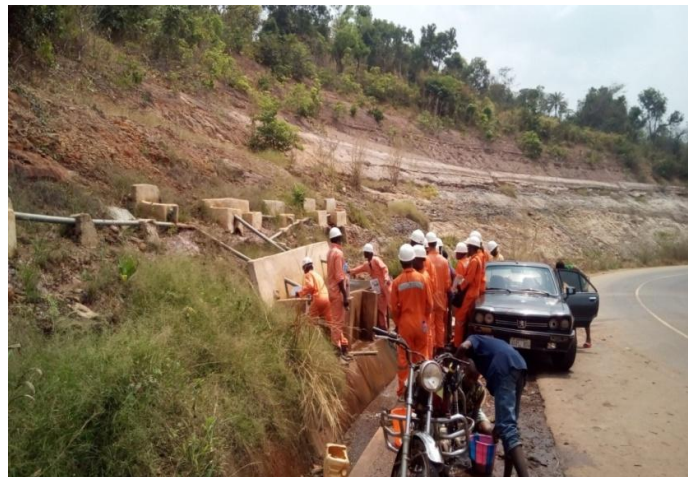
Plate 4. Field photograph showing spring water from the contact between fractured sandstone members of Ajali and Mamu formations, at Agola, west of River Niger
