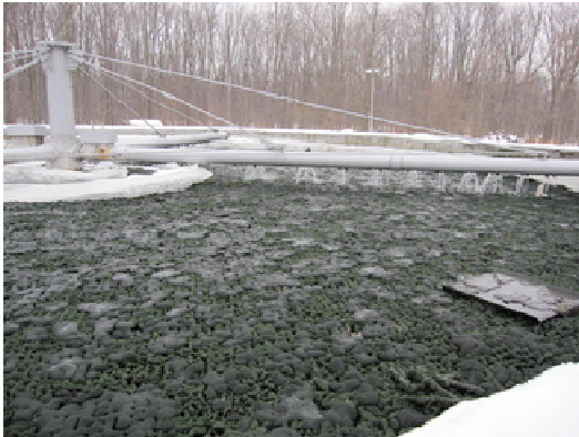
Picture 1. Moss-like species Vaucheria starting to dominate trickling filter [10]
