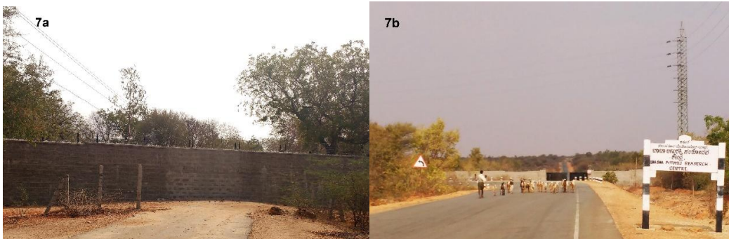
Fig. 7. a) The compound wall built in the Challakere Amrit Mahal Kaval grasslands. b) Bhabha Atomic Research Centre (BARC) agency encroached the village road
